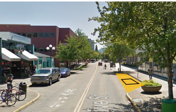
One (1) 7'x20' parking space in front of the UO building at 942 Olive
